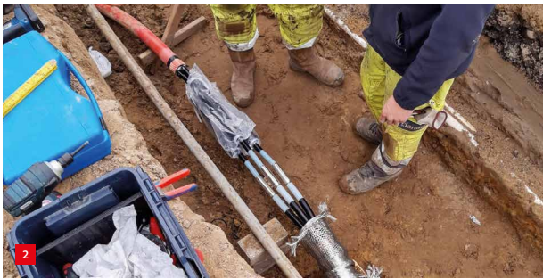
Liander technicians performing cable splicing in the field.
